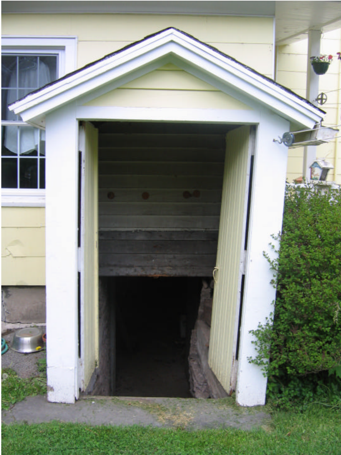
Photo 1 – View from outside looking down stairs
