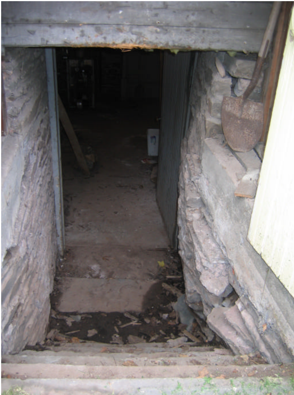
Photo 3 – View looking down stairs
